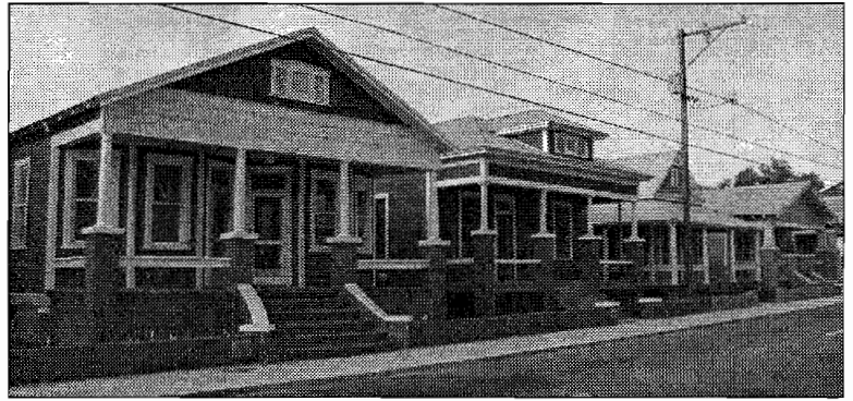
I-4 Historic Preservation Project - Columbus Avenue
